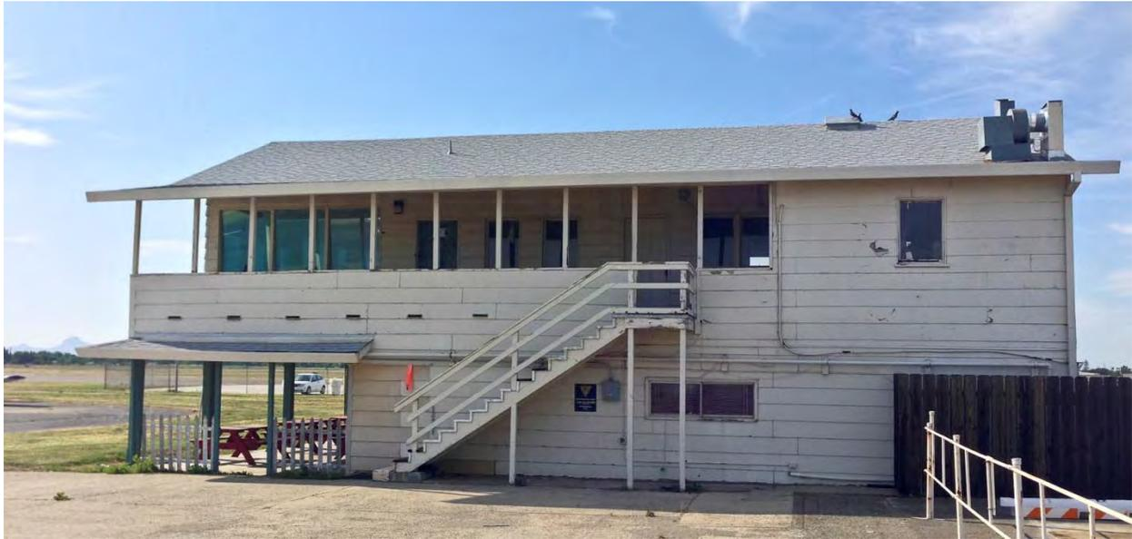
**Figure 4.** *This airport building is in need of paint and maintenance. Airport buildings do not have scheduled maintenance and are now showing signs of wear. The exposed wood and leaking roofs are beginning to require funding and maintenance. Aircraft and equipment are reportedly getting wet in these facilities because of leaking roofs.*
