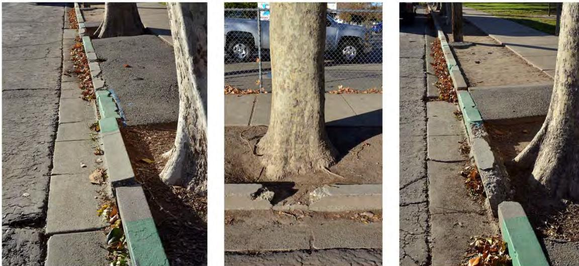
**Figure 3.** *Broken Curbs on the part of 7<sup>th</sup> Street that traverses the Covillaud Elementary campus.*
